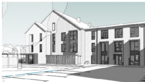
View from the car park of the entrance and bistro
